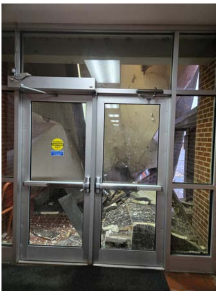
South Entrance Faust Hall
